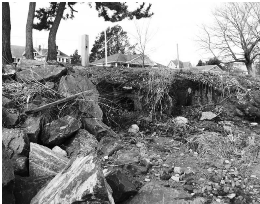
TOP TO BOTTOM: Aerial view of Stillhouse Cove Park and salt marsh; Wenley Ferguson of Save the Bay and Dave Lager, Team Leader at SUMco, assess the damage; and 2012 damage due to Super Storm Sandy.
