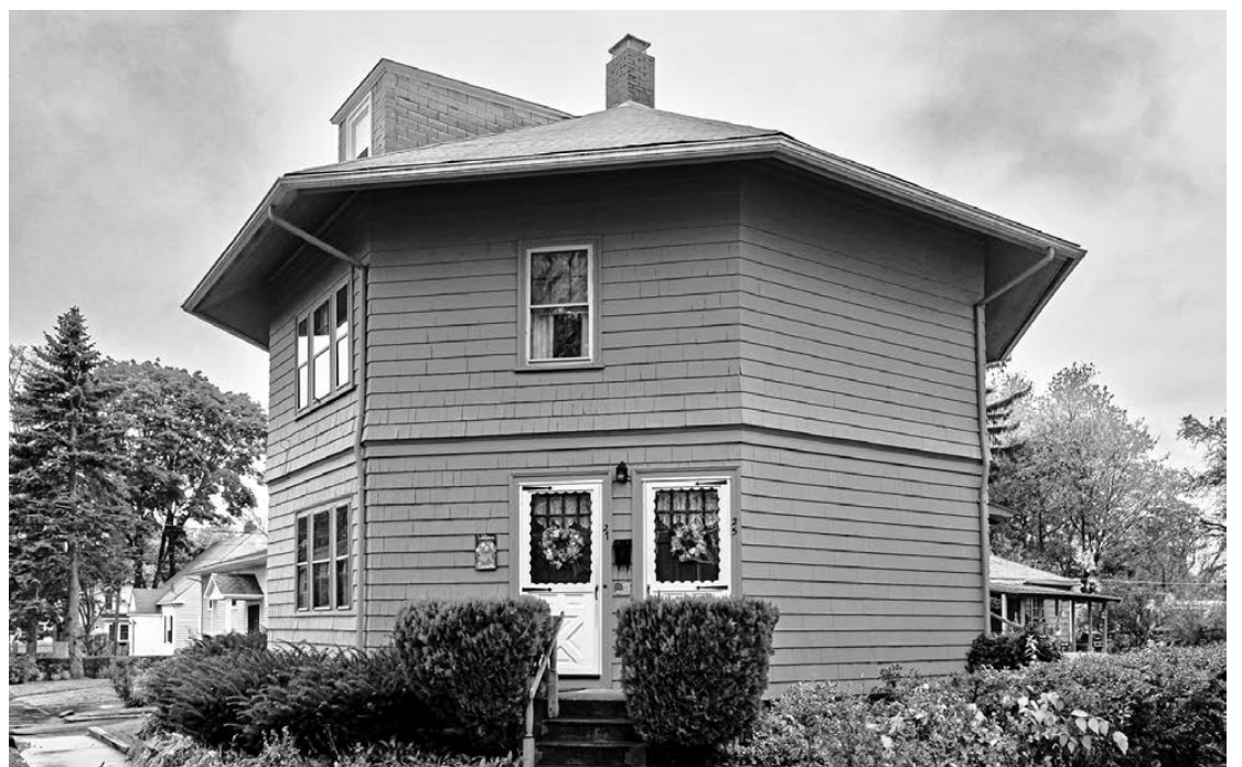
Pawtuxet octagon house at 27 South Fair Street.
